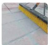
Cleaning of Paver Stone
