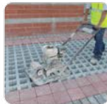
Vibration of Adoquín
